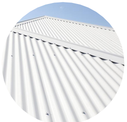
Metal Roof Sheetting (RT-1) Colorbond Custom Orb Roof Sheet (Surfmist)
