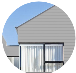
CLD-1 Cladding Type 1 Linea Weatherboard (Dulux 'Dieskau')
